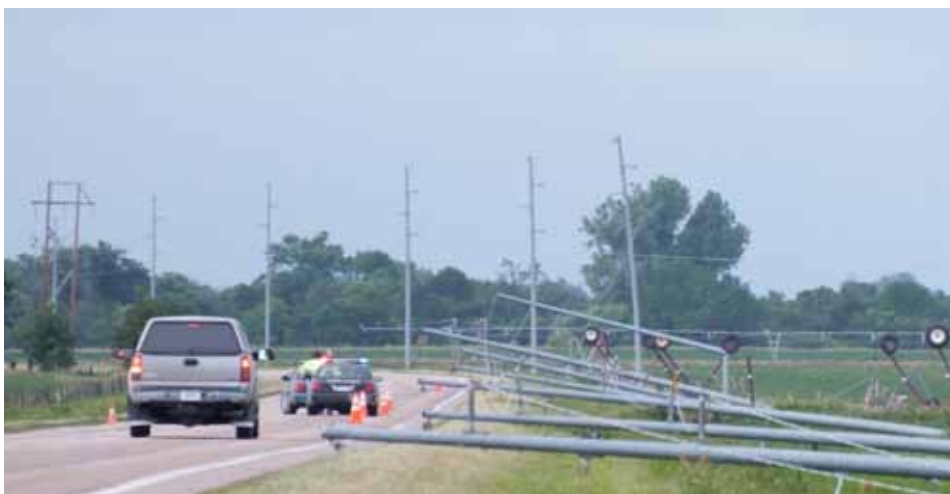
Parts of the steel-pole transmission line along HWY 40 near Amherst were flattened by the storm on June 20. Dawson PPD asks that the public stay away from downed power poles and lines. Lines may still be energized and broken equipment can pose hazards on the roadways.
