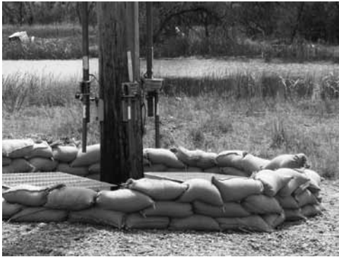
Dawson PPD is monitoring flood conditions along the Platte River and developing contingency plans to ensure we can keep the lights on.
