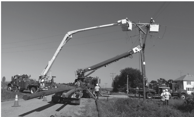
ABOVE: The North Platte construction crew worked with linemen from the Gothenburg Service Center to replace two poles south of Cozad on September 27.
